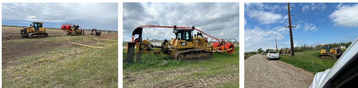
(Above) Construction crews install underground conduit for North Central Communications’ Williston–Williams MVC Project, the largest remaining Capital Projects Fund broadband deployment in North Dakota.
